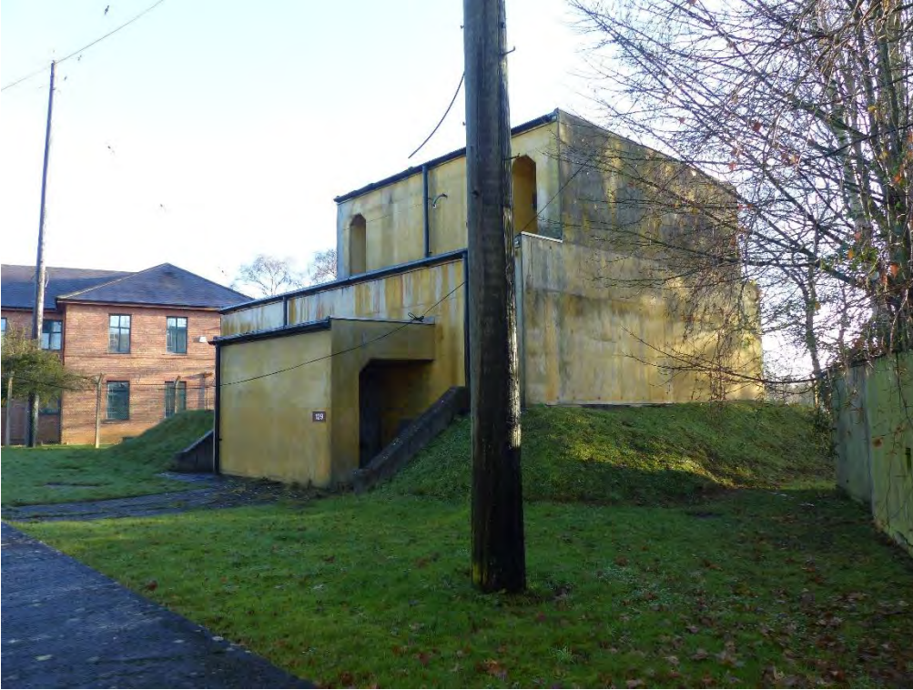
Plate 41: Scheduled Telephone Exchange at RAF Upper Heyford
