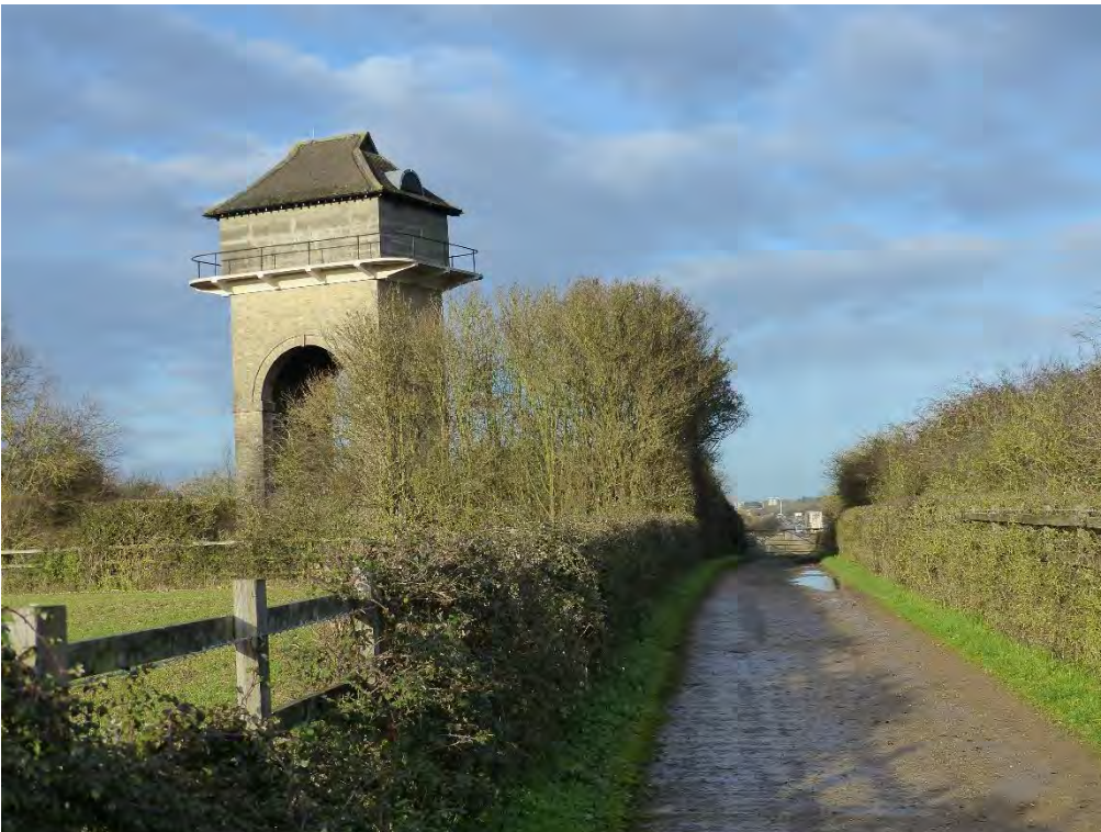
Plate 30: Trow Pool Water Tower, adjacent to M40 (right)
