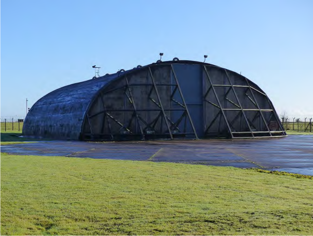
Plate 39: Scheduled Hardened Aircraft Shelter (HAS) at RAF Upper Heyford
