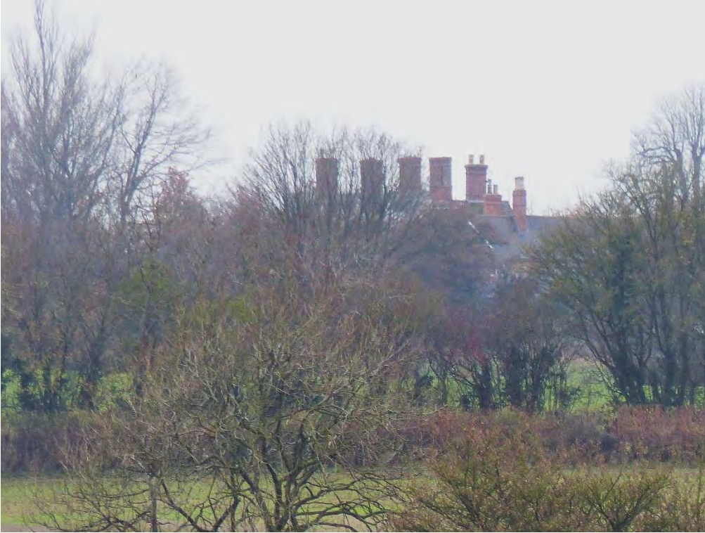
Plate 33: Chimney stacks of Troy Farmhouse, viewed from Area A of Application Site
