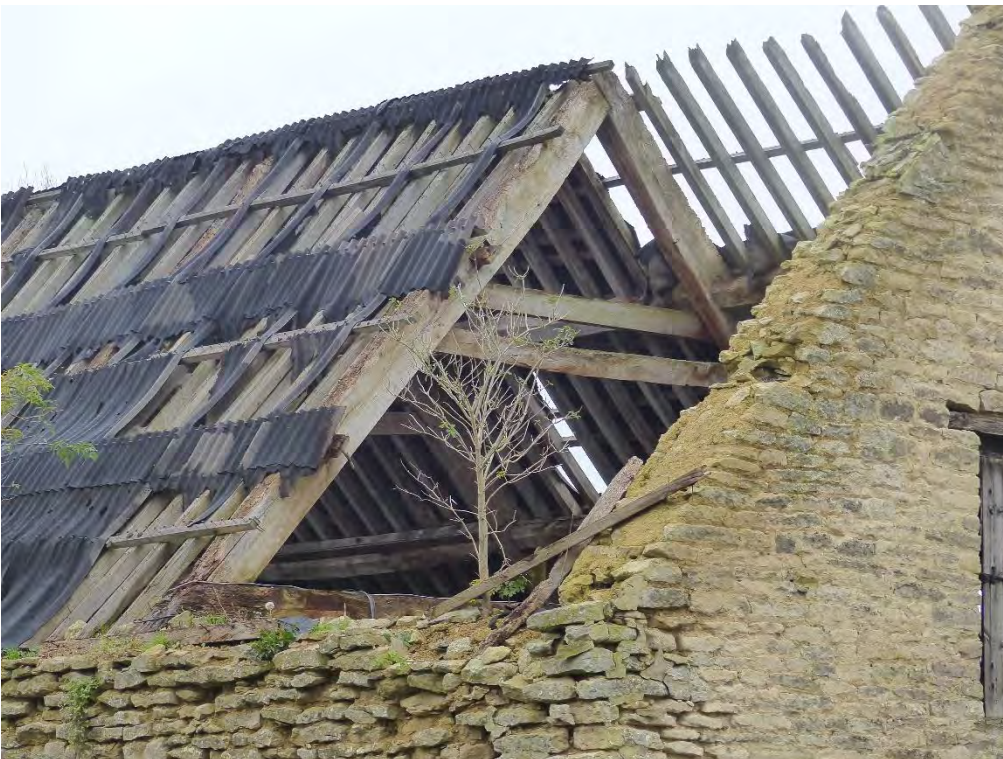
Plate 24: Grade II listed Barn at Ashgrove Farm, roof structure
