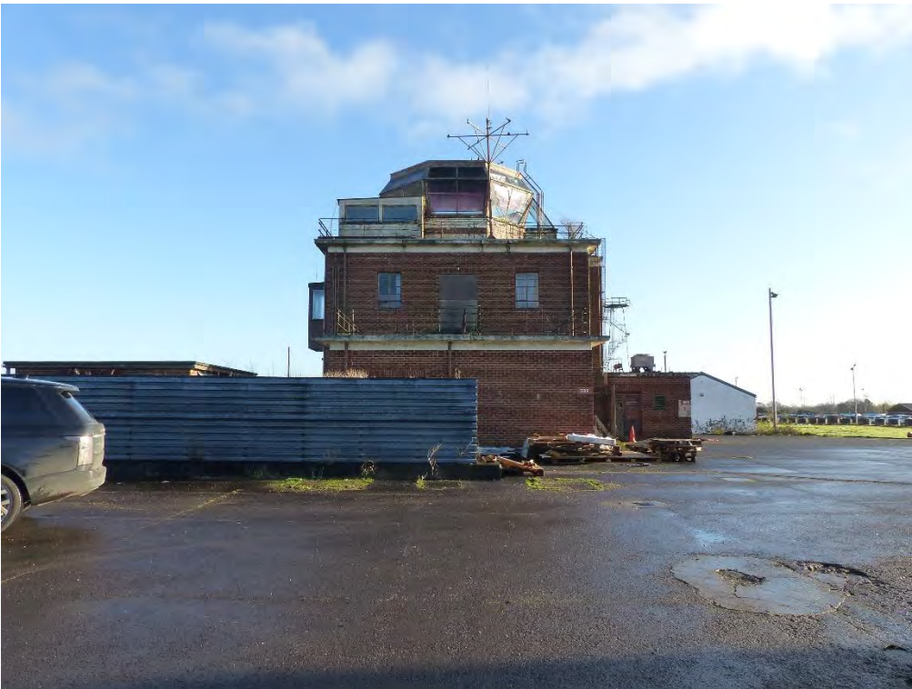
Plate 40: Listed Control Tower at RAF Upper Heyford
