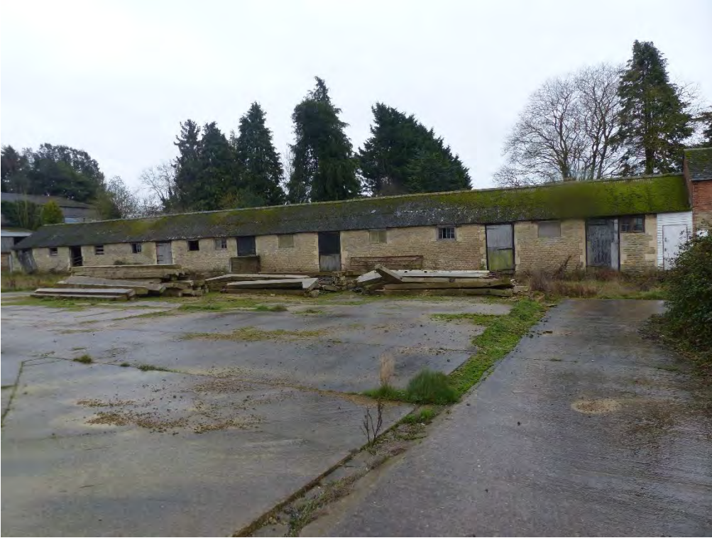
Plate 27: Stable block at Ashgrove Farm, front (north) elevation
