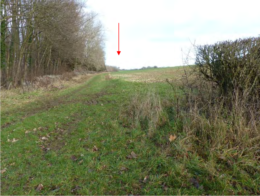
Plate 31: Distant view of Trow Pool Water Tower, from bottom of track leading to Lodge Farmhouse
